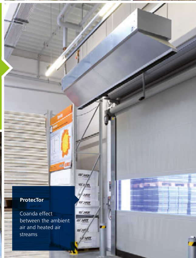
ProtecTor Door air curtain with ambient air and heated air streams for effective screening.
