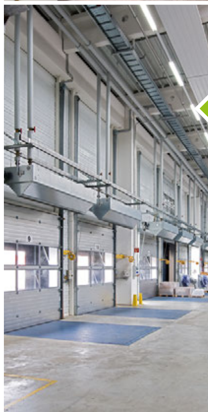
ProtecTor Door air curtain with ambient air and heated air streams for effective screening.
