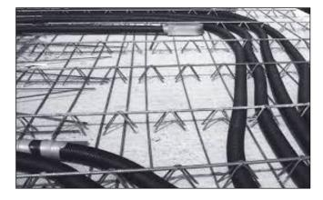
If flexible ducts are inserted into ceilings with fire protection requirements, minimum ceiling thicknesses and/or minimum thicknesses above and below the inserted parts must be take into account. The precise installation situation should be clarified with the local site engineer based on the fire protection concept for the building. Also refer to DIN 4102-4 3.4 Tables 9 and 10.
